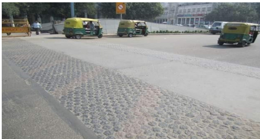
Pic-3: Tabletop with cobble stone on slope and cement concrete surface on top
