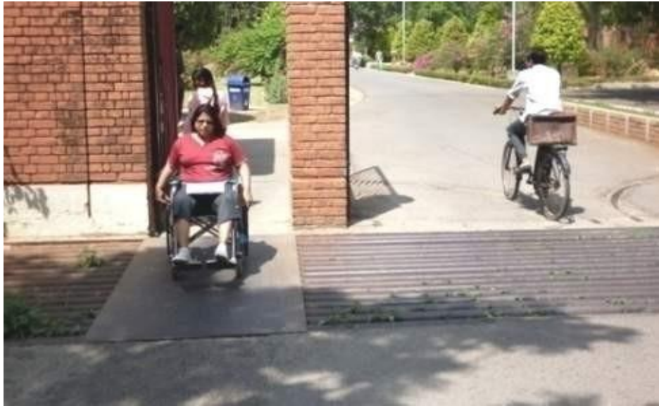
Pic-1: Cow catchers covered with bridge plate
