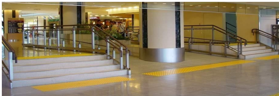
Fig-3: Landings having a row of warning strip
