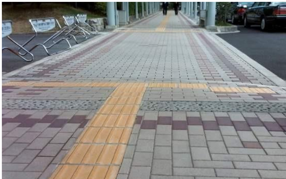
Pic-2: Tabletop with tactile pavers
